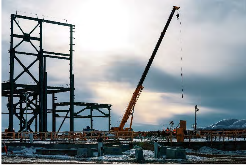
Construction at Great Plains Power Station
